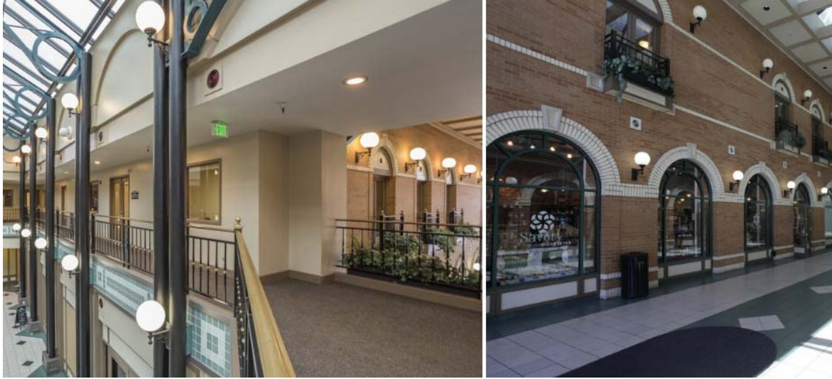
Image 5 123-147 N College Ave Fort Collins, CO 80524 Inside
